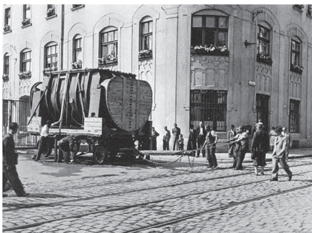
Transport turbogenerators, 1939 rok
