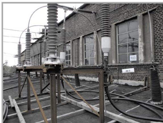
Fig. 8. 110 kV portable cable line usage
