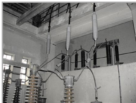
Fig. 8. 110 kV portable cable line usage
