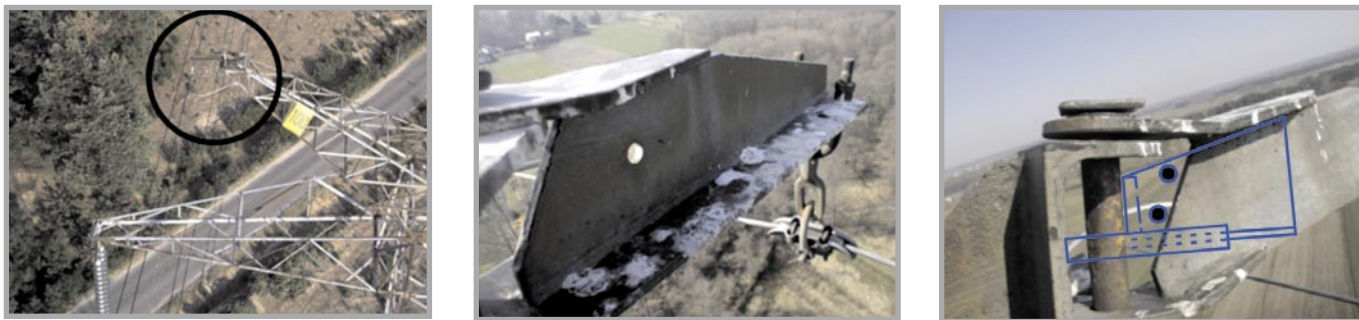
Fig. 5. Installation of lock for swinging suspension on the active power line
